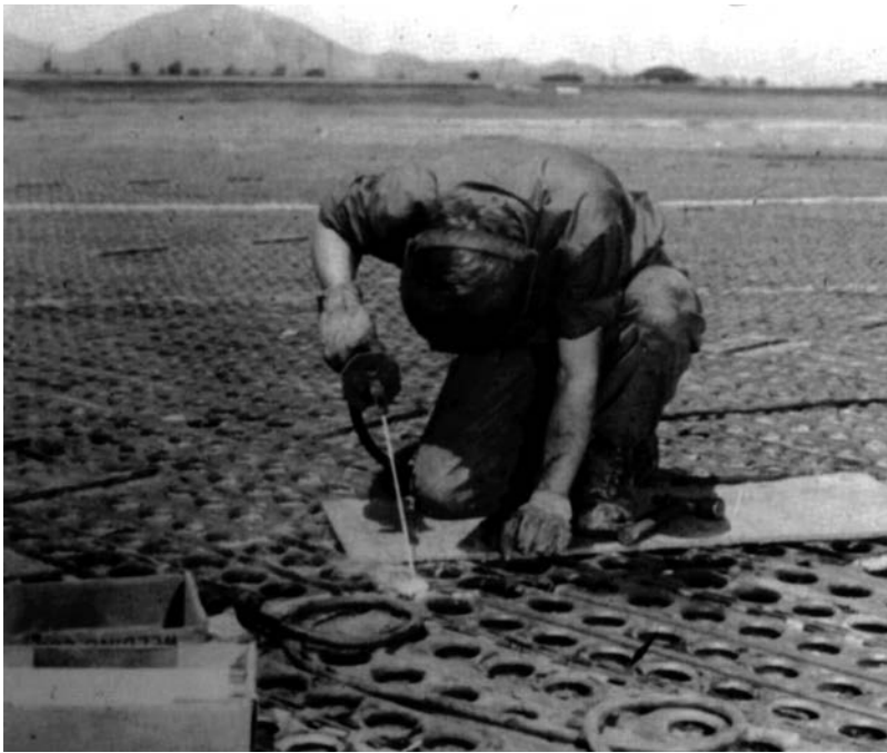
Repairing a pierced-steel planking runway.
