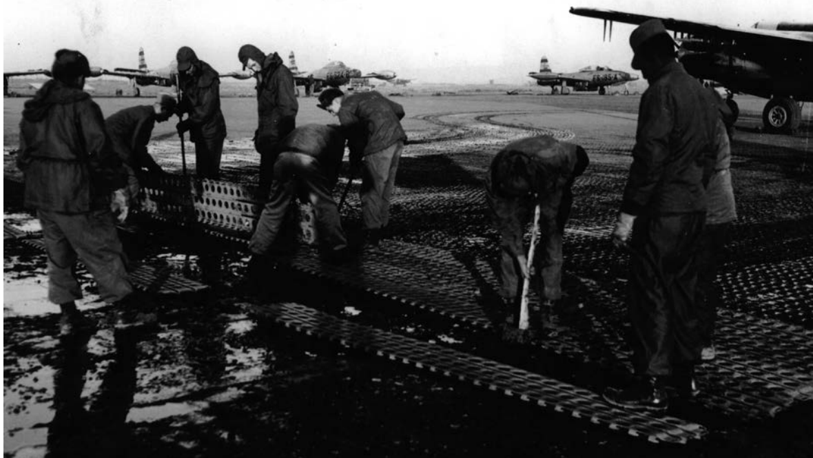
Laying pierced-steel planking over an oiled surface.
