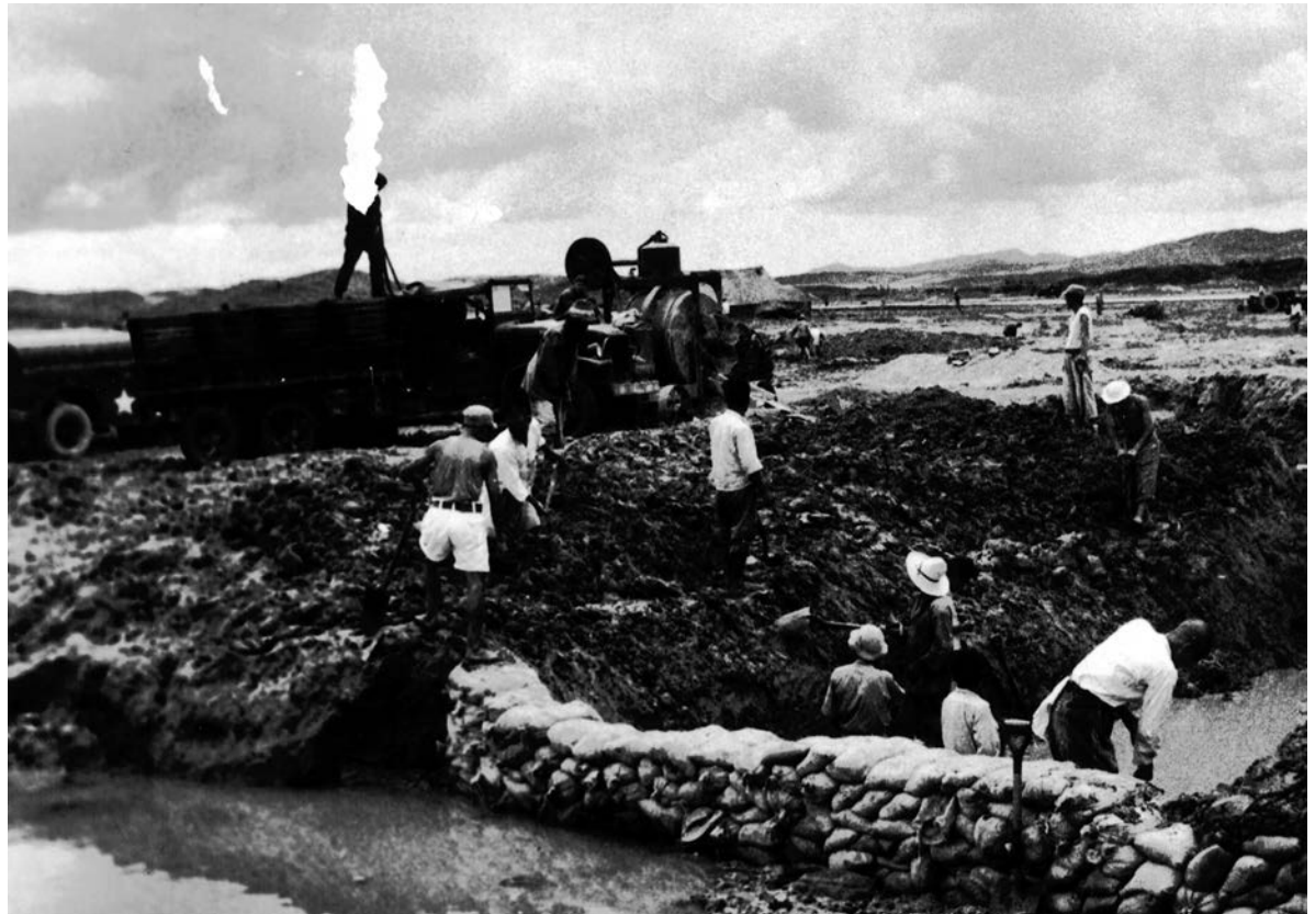
Airfield drainage excavation in Korea.
