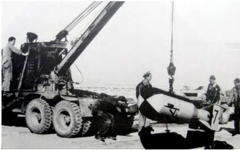
Loading drop test units before the advent of hydraulic lifts. (Photo courtesy of Historic Wendover Airfield.)
