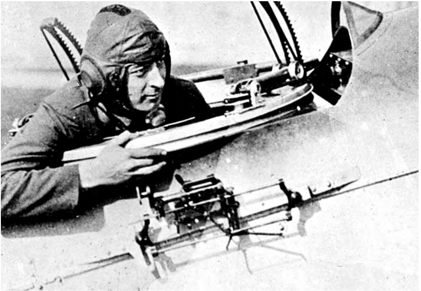
The Drift Bombsight. (USAF photo.)
