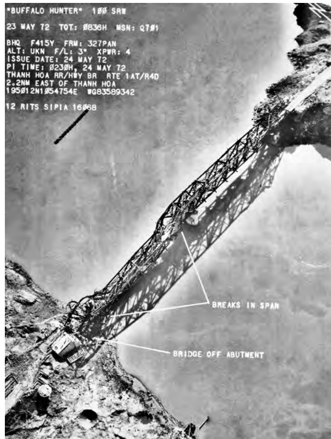
A BUFFALO HUNTER AQM-34 drone of the 100th SRW flew a Thanh Hoa Bridge recce sortie on May 23 on Mission Q701. Damage shown included breaks in the span and the Bridge being off its abutment. According to Col Dick Horne, 8th TFW/DCO, Lt Col Richard Hilton's Goatee flight had been instrumental in the damage to the Bridge.
