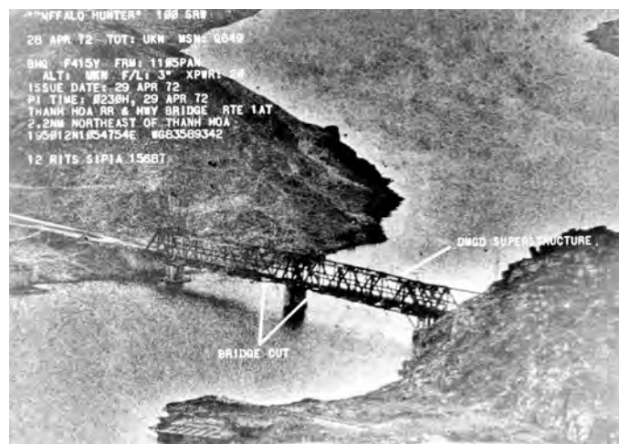
After the April 27 strike against the Bridge, a 100th SRW DC-130 launched a BUFFALO HUNTER drone the next day on Mission Q649 for battle damage assessment: the Bridge was cut and the superstructure damaged. Further photo recce on May 9 showed that it had been completely repaired and serviceable.
