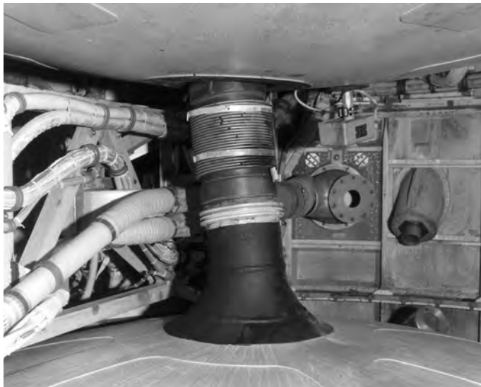
Figure 13: Operation Wrap up. Streaks of corrosion on the top of the Stage II oxidizer tank in the between tanks area of Titan II B-23. Missiles returned during Operation Wrap Up were segregated in a separate factory area where work was conducted around the clock to get the missile tanks and valve joints repaired and the missiles returned to the operational bases. Courtesy Lockheed Martin Astronautics, Denver.
