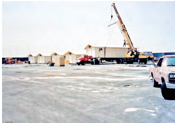
'Shaikh Isa Shacks Moving Day'. The trailers that were used by the 81st TFS as Ops buildings were loaded on flatbeds/eighteen wheelers for transportation to their new home, King Abdul Aziz AB at Dhahran. The Squadron even brought its duty desk along and used it there for life support, helmets, etcetera. [Bart Quinn]
