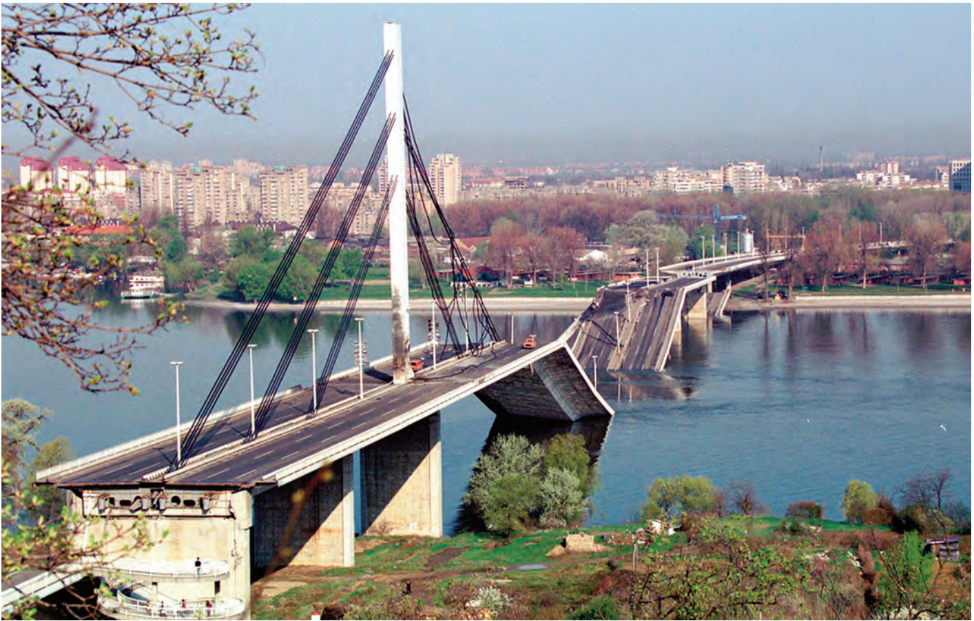
The main bridge over the Danube in the city of Novi Sad, in what is now Serbia, lies broken after NATO bombardment in April 1999. (TASS)
