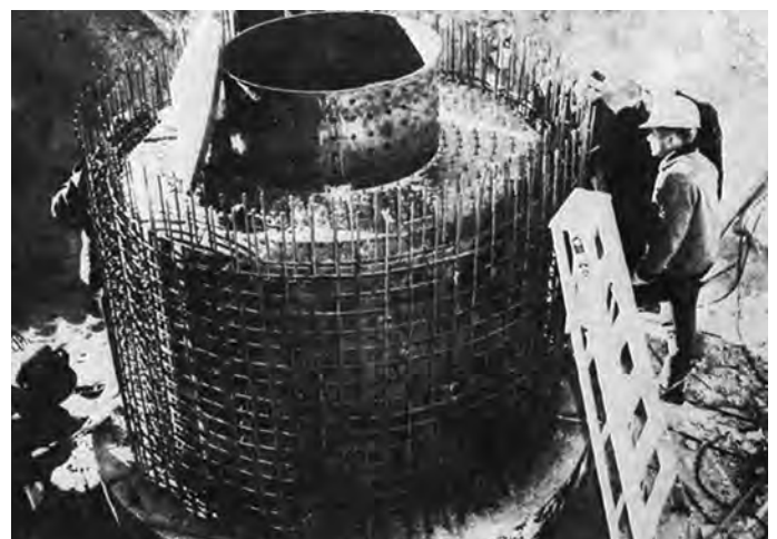
Figure 2. One-fourth scale model of a Minuteman launch facility used in the HEST Phase II experiment.
