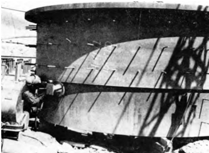
Figure 16. ROCKTEST I. The upper full-scale closure liner for the 30-foot-deep Stub Silo S01. The liner was 7.5 feet tall with an interior diameter of 17 feet and was fabricated from 2-inch-thick steel. The walls of S01 were 5-feet thick. The closure doors were cast in place.
