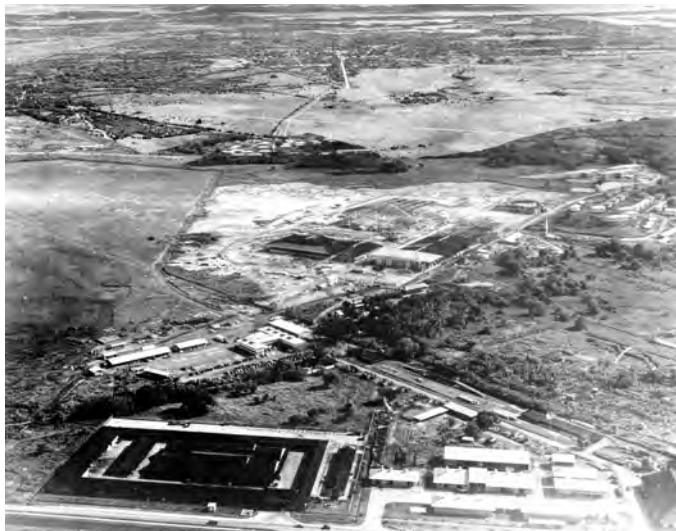
Work on the Panama Air Depot started in April 1940, with some buildings completed by March 1941. This June 1941 aerial photo of Albrook Field shows major construction work under way. (US National Archives.)
