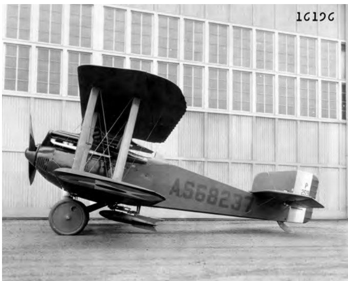
The Boeing MB-3A was the first true pursuit aircraft assigned to the 24th Pursuit Squadron. As seen here, the aircraft could be fitted with a bomb rack and used in the ground attack role. (US National Archives.)
