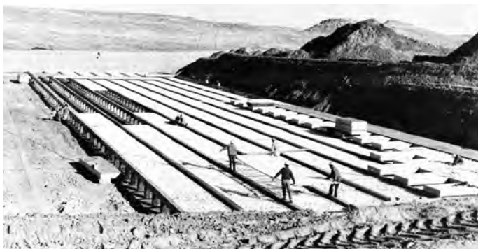
Figure 7. HEST-I. Workers are laying out the floor before installing the frames with Primacord. (Courtesy of Boeing Company.)
