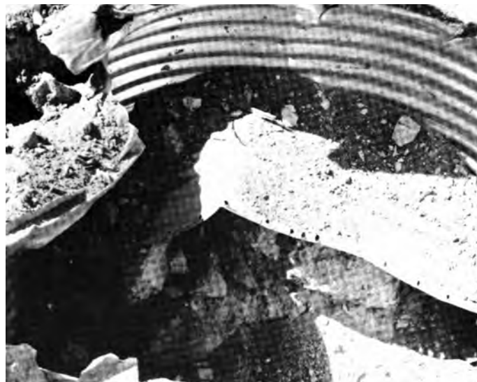
Figure 15. DATEX II. Close up of the top of Structure S3. S3 was 6 feet in diameter and 15 feet deep with a liner consisting of a 6-foot diameter section of steel culvert backfilled to the rock walls with approximately 9 inches of non-reinforced concrete. The top 5 feet was sheared off the silo and moved 13 feet laterally. The lower portion of the silo also moved approximately 6 inches laterally.
