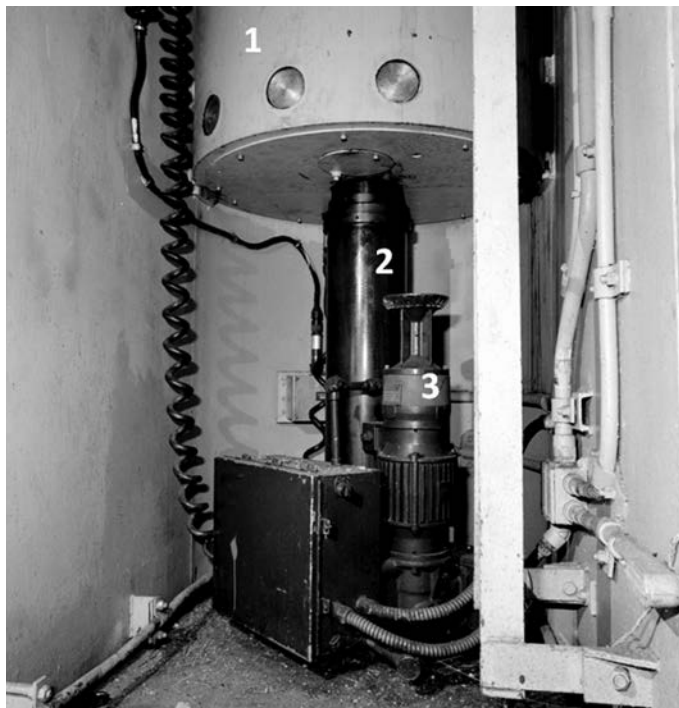
Secondary door fully retracted, Launcher Equipment Room Level 2: 1) 4-inch diameter locking bolts; 2) linear actuator; 3) manual override drive for linear actuator. (Library of Congress)
