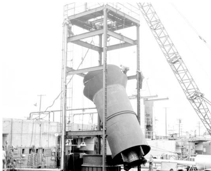
Figure 21: (Above) Construction of the Silo Model. The launch duct and exhaust ducts were installed in one piece. Courtesy R. Pickford.
