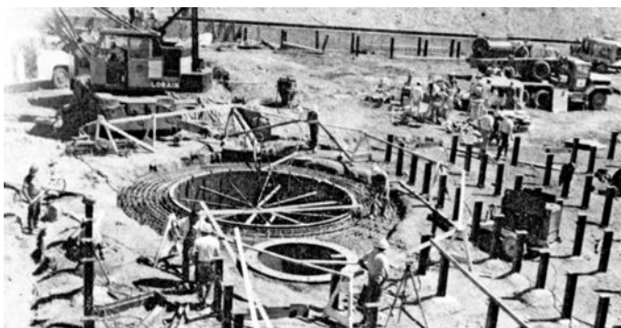
Figure 17. ROCKTEST I test facility under construction. The large diameter circle is the top of 30-foot-deep stub silo wall. The full-scale closure liner has not been installed. The smaller diameter circle is an access tube for post-test inspection of the closure.
