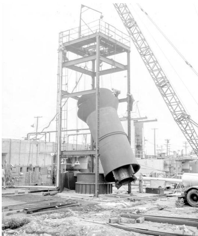
Construction of the 1/6th scale Titan II in-silo launch test facilities at Aerojet, Azusa, California. The facility was built and the testing completed in a 60 day period. Aerojet opted for a W-shaped deflector with cascade vanes to direct exhaust away from the silo opening, preventing entrainment of exhaust products. (Courtesy of Rollo Pickford)
