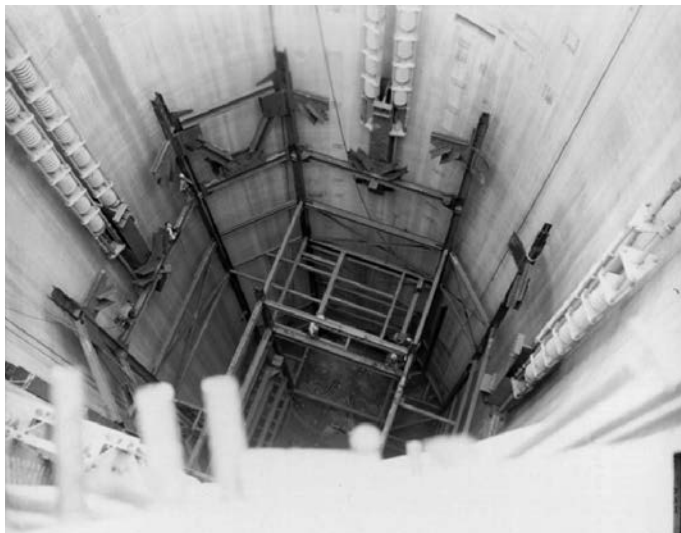
(Above) Atlas F: Upper wall bracket for crib shock isolation system. The point of attachment was at Level 2. The bracket was over 6 feet tall ( Atlas-missilesilo.com ) (Below) Atlas F: Lower crib shock isolation system bracket attachment to crib structure at Level 6. Note the workers on the beam below the leftmost spring set. ( Defense Visual Information Distribution Service )
