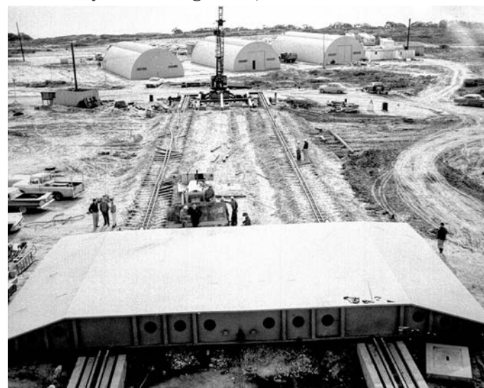
Figure 27: Silo Closure Door at Launch Facility 395-B, Vandenberg Air Force Base. The silo closure door was assembled as close to the launch duct as feasible. Here the door is being moved to Site 395-B. Author's Collection.
