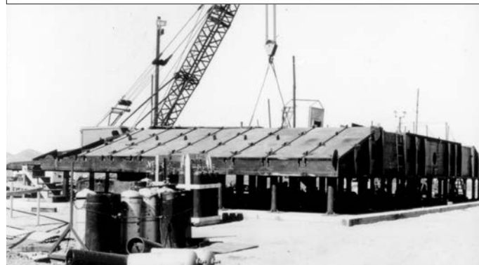
Figure 26: Silo Closure Door Detail. Upper: Diagram illustrating the "eggcrate" construction of the massive 700-ton silo closure door. The top and bottom plating was 3.5-inch battleship armor. The interior webbing supports varied from 1.375 inches to 2.5 inches in thickness. Lower: The silo closure door was prefabricated in sections and assembled on site. The pedestals will be removed and the door lowered onto temporary rails for movement onto the silo. Courtesy Titan Missile Museum Archive.
