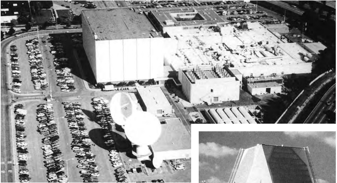
(Above) The "Blue Cube," Onizuka AFB, California. (Far right) Pave Paws radar installation.
